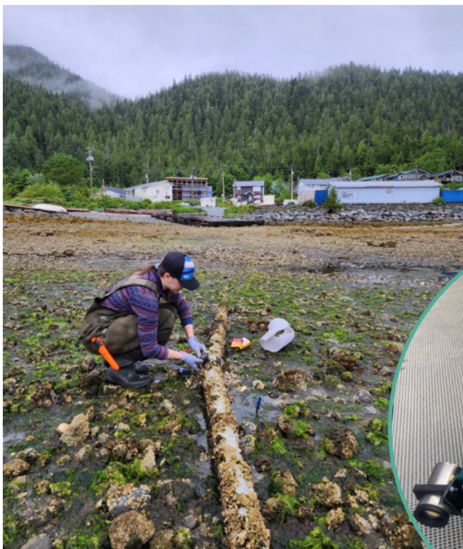
Above: Jr. project engineer Miranda Herle installed subsea cable protection for the Hartley Bay cabled coastal ocean observatory. Inset: Hartley Bay observatory.
